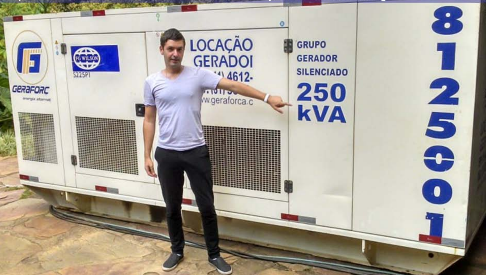
Boris Petrovic – With the needed 250kVA generator
